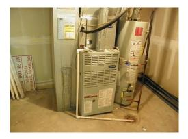
**Description:** Model 58PAV111-16, Carrier forced air natural gas furnace. The unit has an input rating of 110,000 BTU/hr. output rating of 89,000 BTU/hr., and maximum outlet temperature of 185°F.
