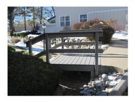
**Description:** The bridge is built with Trex® floor boards and railing. The decking has an under-structured wood frame with an estimated 390 square feet of Trex® deck boards and Trex® built-in benches.
