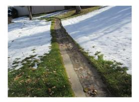
**Description:** The onsite drainage systems within the community utilize grass and cobblestone swales, sloped grade, area inlets, sidewalk chase drains, and concrete drain pans to convey surface runoff to the public storm drainage systems.
