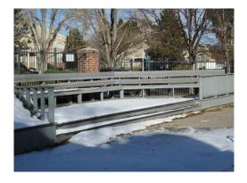
**Description:** The bridge is built with Trex<sup>®</sup> floor boards and railing. The decking has an under-structured wood frame with an estimated 390 square feet of Trex<sup>®</sup> deck boards and Trex<sup>®</sup> built-in benches.
