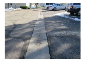
**Description:** Estimated 15,182 square feet of concrete drain pans. The drain pans on site were 1- to 3-foot wide and presumed to be on-grade and reinforced. Several drain pans on site were attached or adjacent to walkways.
