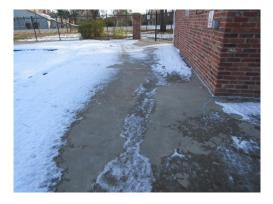
**Description:** Estimated 4,705 square feet of concrete pool deck that is cast-in-place, ongrade, reinforced, concrete slab.
