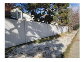
**Description:** Estimated 2,375 linear feet of white vinyl fencing intermittent between 1,056 square feet of brick veneered columns.
