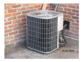
**Description:** Model 38CKC, Carrier Weather Mate Series air conditioner. The air conditioner has a seasonal energy efficiency ratio of 11.5.
