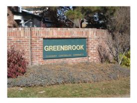
**Description:** Estimated 735 square feet of CMU walls covered with an estimated 1,575 square feet of brick veneer that frames three rectangular, painted concrete signs with lettering attached.
