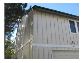
**Description:** Estimated total of 194,201 square feet of vertically-orient, channel board siding. The trim around the windows and at corners is installed on the top of the siding boards. Lap siding is installed in the horizontal direction for the Phase 2 patios.
