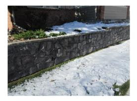
**Description:** Estimated 157 linear feet of adhered, natural stone veneer, with grouted mortar joints.
