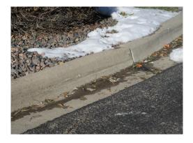
**Description:** Estimated 6,469 linear of 6-inch vertical face curbs with 12- to 24-inch wide concrete gutter sloped in a catch or spill position.
