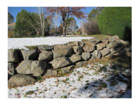
**Description:** Estimated 2,017 linear feet of stacked boulder retaining walls at a range of 1 to 4 feet in height.
