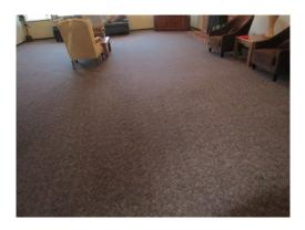
**Description:** The majority of the flooring for the interior common areas is finished with commercial grade carpet, estimated at 1,311 square feet. The upper level bathrooms and kitchen is finished with brick tile flooring, estimated at 264 square feet.
