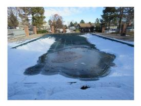
**Description:** Estimated 3,188 square feet of swimming pool surface. The swimming pool is finished with a cementitious plaster basin. The pool coping appears to be colored and stamped concrete product integral with the pool deck.
