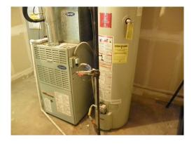
Description: Model PR640, State Select automatic storage water heater. The water heater has a 40 gallon capacity with an input rating of 40,000 BTU/hr.
