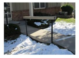
**Description:** There is a combination of metal and wood handrails supported by metal posts that are fastened to concrete walks or ground packed.
