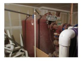
**Description:** Model HRL-48, Swimquip sand filter. The filter has filtration area of 12.6 square feet and a design flow capacity of 15 to 20 gallons per minute.
