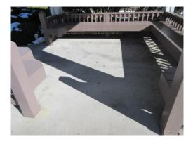
**Description:** Estimated 504 square feet of concrete slabs that are assumed to be ongrade and reinforced.
