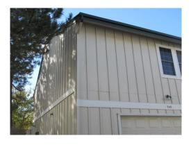
**Description:** Estimated total of 194,201 square feet of vertically-orient, channel board siding. The trim around the windows and at corners is installed on the top of the siding boards. Lap siding is installed in the horizontal direction for the Phase 2 patios.
