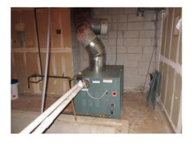
**Description:** Model WH-970, Parker Boiler Company gas fired boiler assembly.
