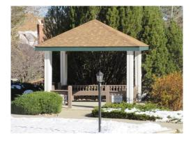
**Description:** Asphalt shingled roof structure with wood trim and fascia supported by four wood posts. The interior of the gazebo area contains built-in wooden benches.
